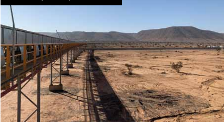
The whole conveyor was completed in two months
