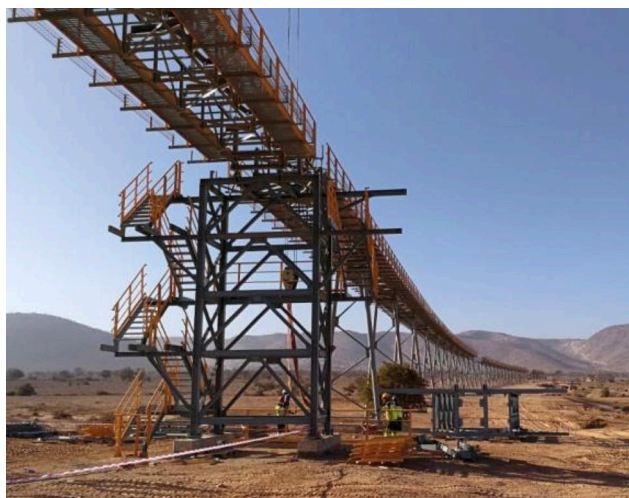
Figure 1. Lafarge long-distance belt conveyor during erection.
