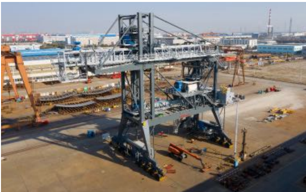
Figure 1. Cargill shiploader in erection phase.
