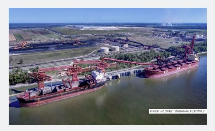
To Convent Marine Terminal coal yard in Louisiana, US, Bedeschi supplied three shiploaders with radial-tower type loading booms and two connecting conveyors. The shiploaders are designed to operate at a maximum rate of 6,000tph each. This maximum combined loading rate can be achieved by operating one or a combination of the three shiploaders. All of the conveyors have been designed for a 84in belt. The link belts are also rated for 6,000tph with 84in belts.
