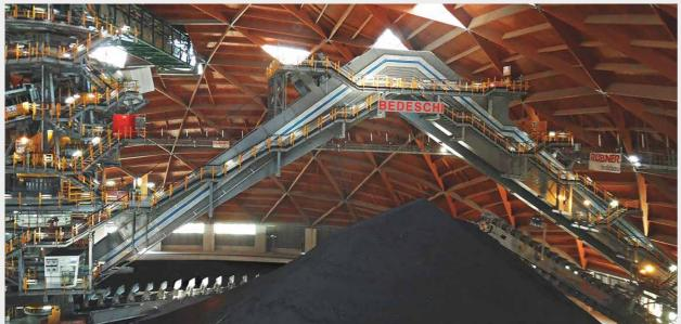
Bedeschi supplied Enel with 2 circular storage in 2011; the Group completed the automation of the Federico II bunker, in Brindisi (IT). The project, one of the most innovative in Europe, consists of 2 indoor domes completely computerized for the storage and reclaiming of coal, feeding the whole plant.
